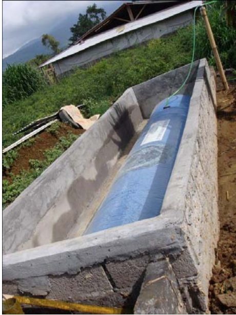
Biodigester used in the Bali Biogas Program
